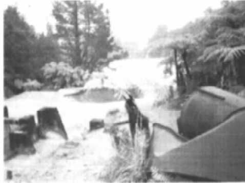
Looking from further up, some of the machinery and hoppers till around with the remnants of 44 gallon drums and such like. The sterile tailings area can be seen in the back ground.
